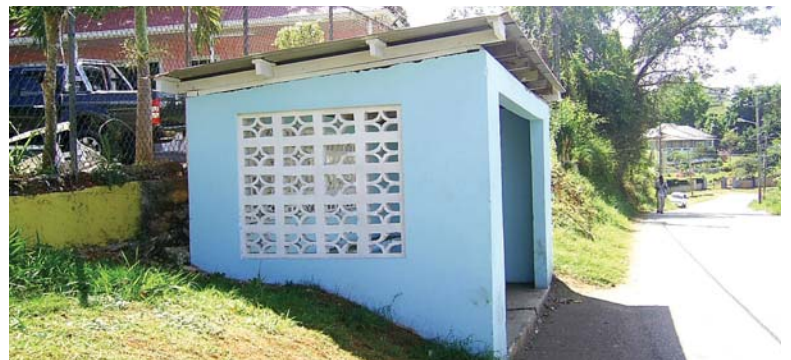
One of several bus stops painted and roadways bushed in December.
